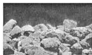
FIG. 5. DEMOLITION WASTE BEFORE PROCESSING
