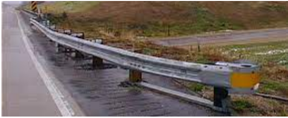
(c) End Treatment (Trailing Side) A Trailing Terminal (TT) arrangement is recommended for the departure sides.
