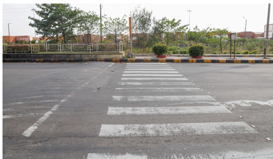
Inaccessible Pedestrian Crossing
