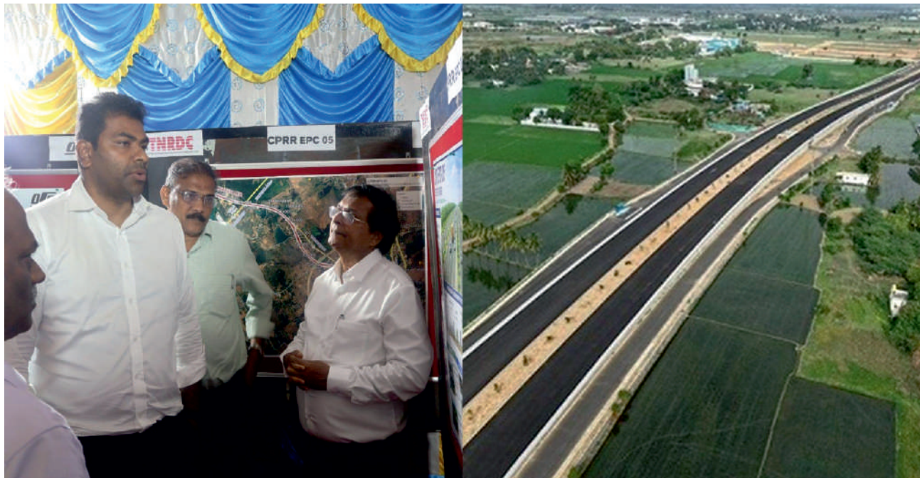
The Hon'ble Minister for Public Works and Sports Development inspected the Chennai Peripheral Ring Road Project in Tiruvallur District on 17.07.2026.
