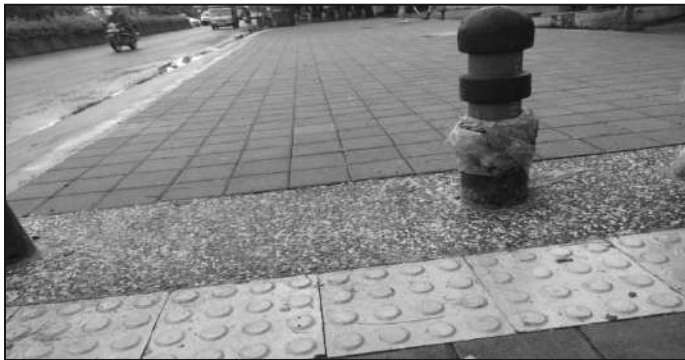
Photo 35 Special Type of Chip Finishing for Fixing of Concrete Bollards in Rectangular and Uneven Areas
