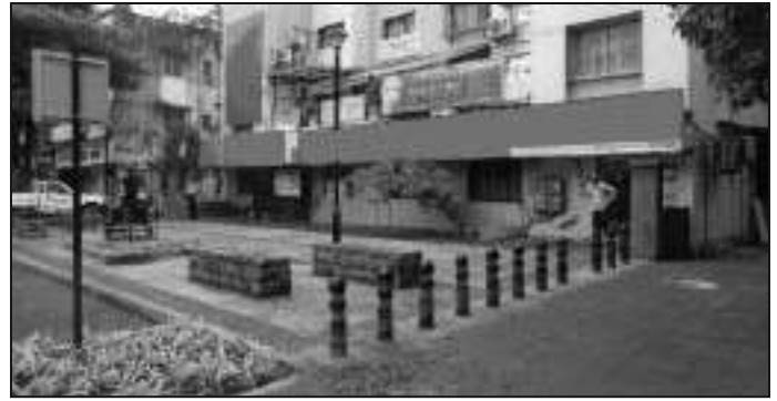
Photo 25 Completed Footpath with Street Elements
