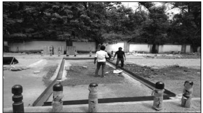
Photo 48 Use of Steel Frames for Raised Pedestrian Crossings to Avoid Paver Block Movement under Traffic
