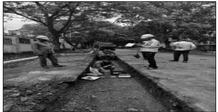
Photo 51 Compaction Density Checking for Utility Backfill and Footpath Portions
