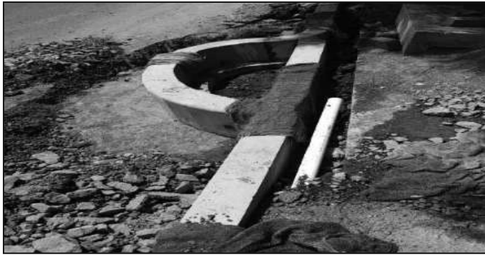
Photo 33 Fixing of Specially Cased Heavy-duty Kerbs for Footpath and Soft Areas
