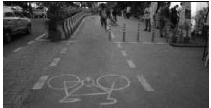
Photo 40 Pedestrian Walkway and Cycle Lane Marked with Temporary Paint for Mock trial
