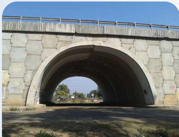
TechSpan® for CUT'N'COVER ARCHES 2010 - Bhandara Bypass, Maharashtra
