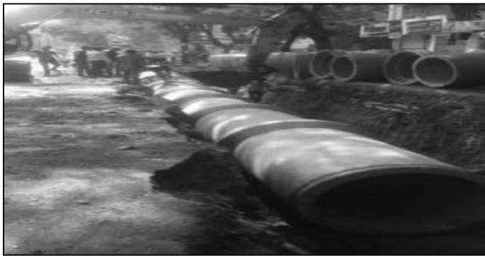
Photo 45 Laying of Storm Water Line with RCC Chambers along Edge of Main Carriageway
