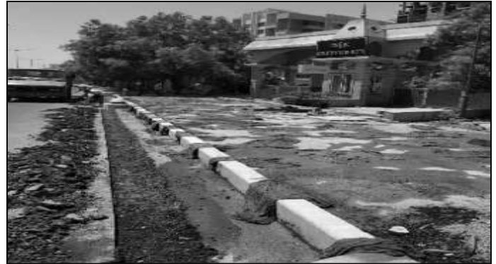
Photo 47 Meticulous attention to Work Quality and Construction Process Like Curing of Joints between Kerbs
