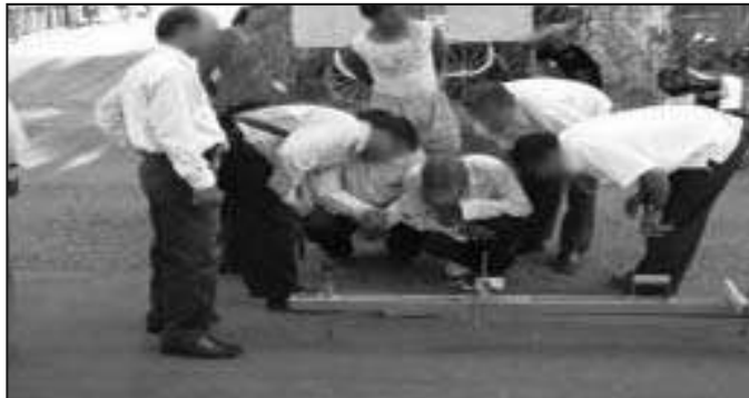
Photo 30 Benkelman Beam Deflection Test for K value Determination before Overlay
