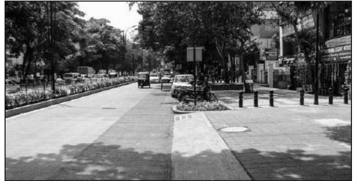
Photos 28 and 29 - 4 Lane Carriageways with Provision of 6.0 m Wide Concrete White Topping Overlay as Carriageway on Both Sides and 1.8 m Paint Marked Cycle Lane
