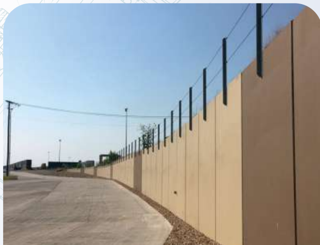
TechWall™ for RETAINING WALL APPLICATIONS 2017 - Pacific Mesquite Expansion Design-Build, Texas
