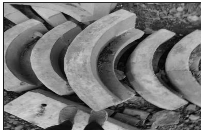
Photo 32 Various Shape and Sizes of Semi-Circular Prestressed Concrete Kerbs Designed and Factory Casted for Project
