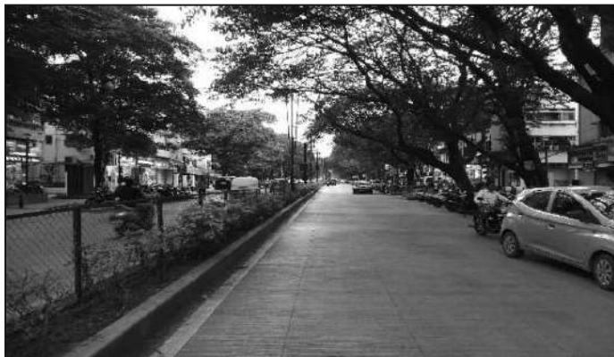
Photo 6 Divided Carriageway with 6 m Width on each Side of Median (3 m Wide Lane)
