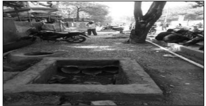
Photo 42 Chambers at Regular Intervals of 25 to 30 m for DWC Pipes and Individual Property Connections from Chamber
