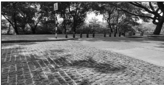
Photo 36 Cobble Stone Finishing used as a Traffic Calming Measure near Pedestrian Crossings
