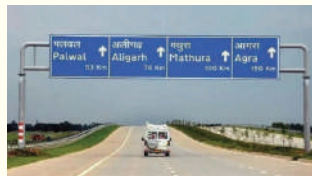
GANTRY & CANTILEVER BOARD
