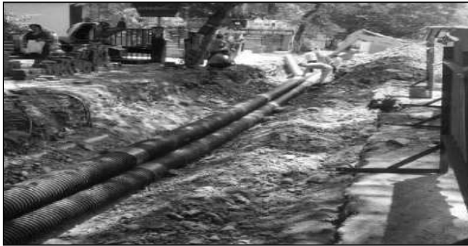
Photo 41 Laying of Double Wall Corrugated (DWC) Pipes 3 Rows for OFC Utilities
